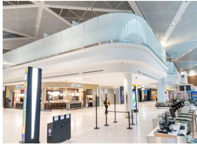
Freestanding Railings: Used curved gradient glass and structural steel supports.
