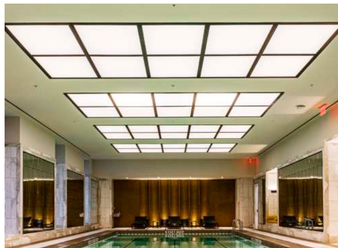
Large Light Boxes: Integrated LEDs illuminate pool areas.
