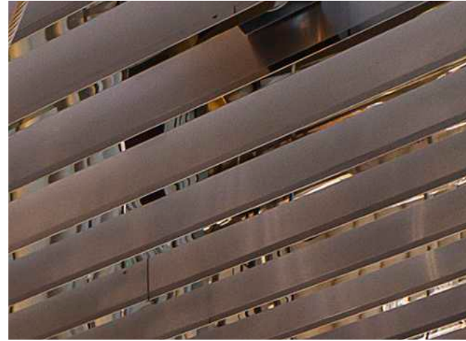
Dual-Finish Metal Fins: Provided visual depth with polished and brushed surfaces.
