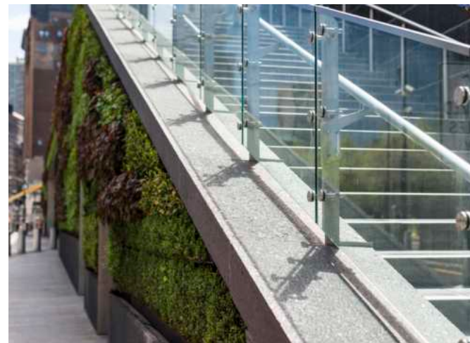
Laminated Glass Technology: Provided both safety and aesthetic appeal in high-traffic areas.
