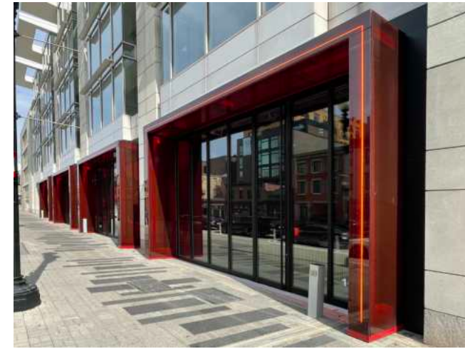
glassXL Panels: Full-height, oversized structural glass for curtain wall façades.
