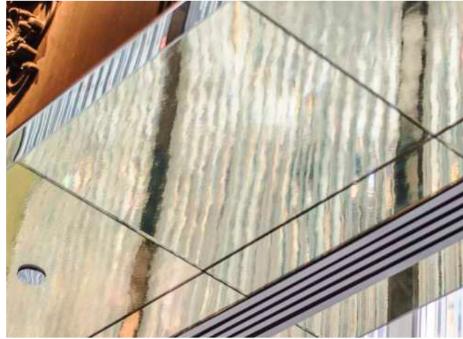
Invisible Mirror Attachments: Luxury mirrors installed with hidden fixtures.
