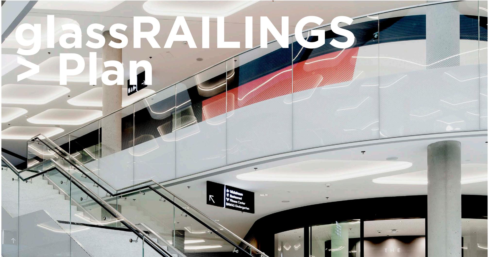
CARVART's new innovative interior and exterior glassRAILING system features a **completely flush, structurally glazed** product that **conceals all attachment methods**. With **no visible hardware**, the glass provides **elegant** and **seamless** lines.
